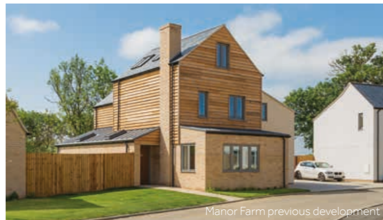
Manor Farm previous development
